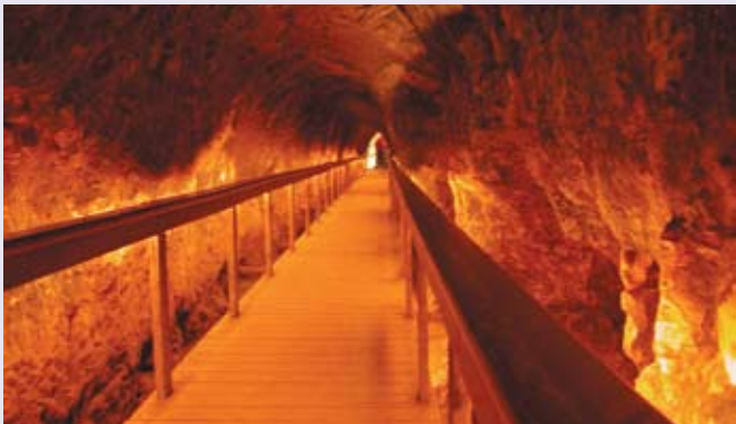
The horizontal tunnel of the water system
